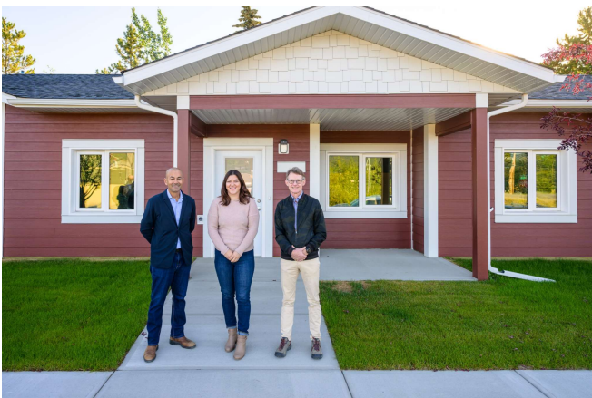
The opening of the Whitehorse Rapid Housing Initiative Triplex at 2 Sycamore Street alongside Minister Ranj Pillai and Whitehorse City Councillor Michelle Friesen, August 2022
